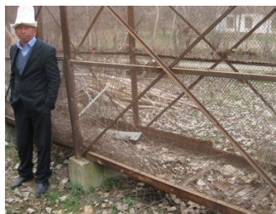
Figure 10: “Drying race” now dilapidated. Used to dry 100 tonnes per season.
