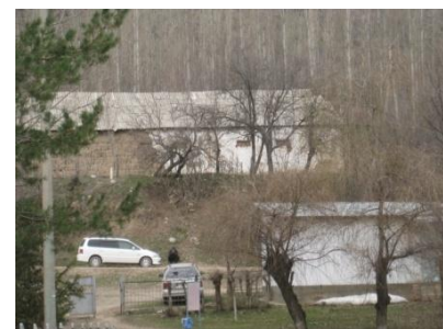
Figure 11: Leskhoz storage building (in background).
