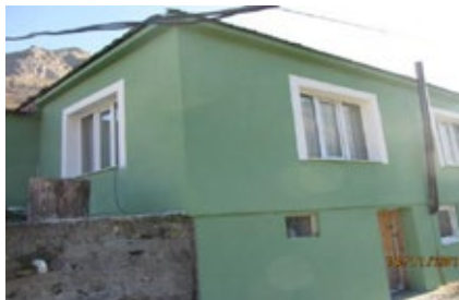
Exterior thermal insulation
