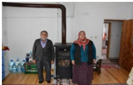
Central heating system for households
